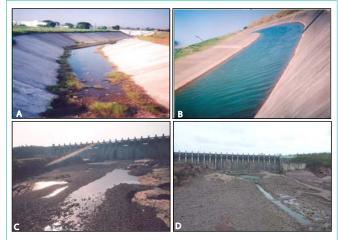
Figure 1A: Indira Sagar Canal before implementing mitigation measure. Figure 1B: After Cleaning and deweeding of canal. Figure 1C: Indira Sagar Dam-Downstream flow of seepage water. Figure 1D: Channelization of water to provide a constant flow.
