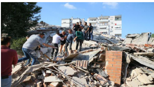
Figure 15: Earthquake caused structural damage.
