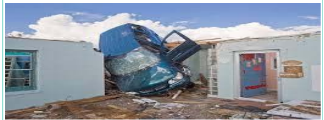
Figure 5: Damage caused by Tornadoes.
